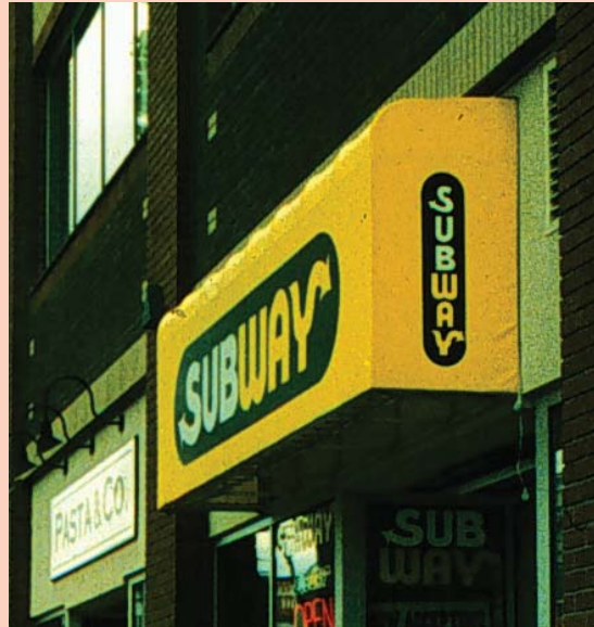
This awning does not cover the sidewalk enough to offer effective protection for pedestrians.
