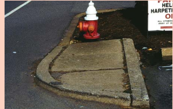
Not only is this sidewalk not continuous, it is too narrow and offers no buffer between pedestrian and the street.
